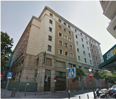
Before office building
