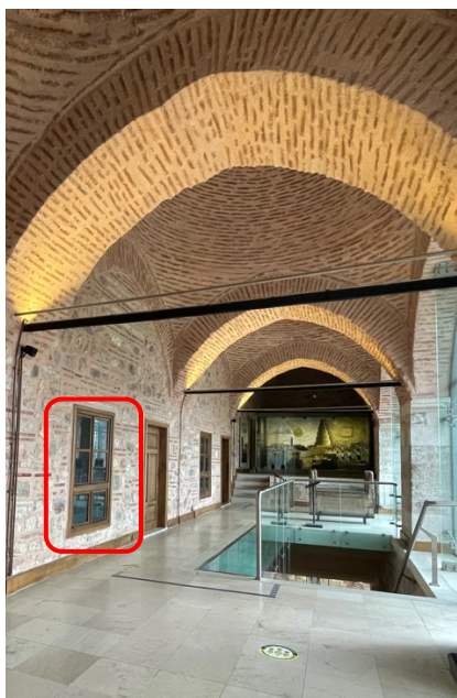
Figure 174. A view of the corridor of TIEM in 2021. The red rectangle indicates the window, which is a display niche. Source: Photo was taken by the author, 2021.
