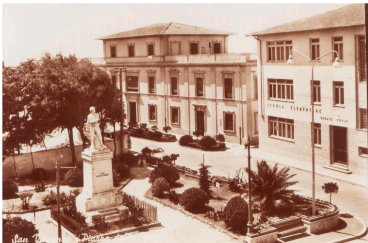
Figure 93 - The ex-CDF of San Vincenzo as an elementary school. Source: http://san-vincenzo-foto-storiche.blogspot.com/2009/09/170-piazze-centrali-20.html
