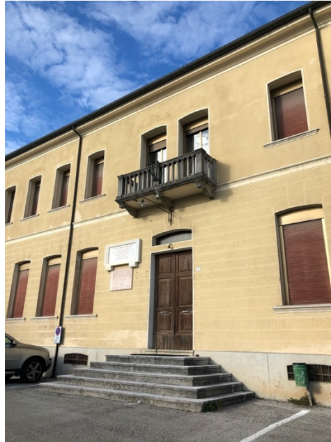
Figure 114 - The facade of the ex-CDF with the plaque of Mussolini speech and economic sanctions. Source: photo of the author.
