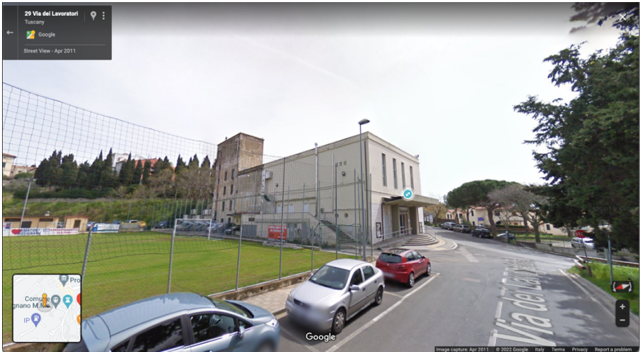
Figure 77 - The ex-CDF, now Municipality of Rosignano and cinema. View from the football field. Source: Google maps
