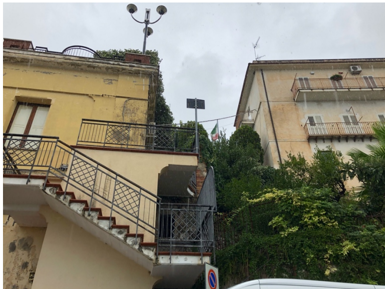
Figure 55 - The stairs of the ex-CDF. Source: photo of the author.
