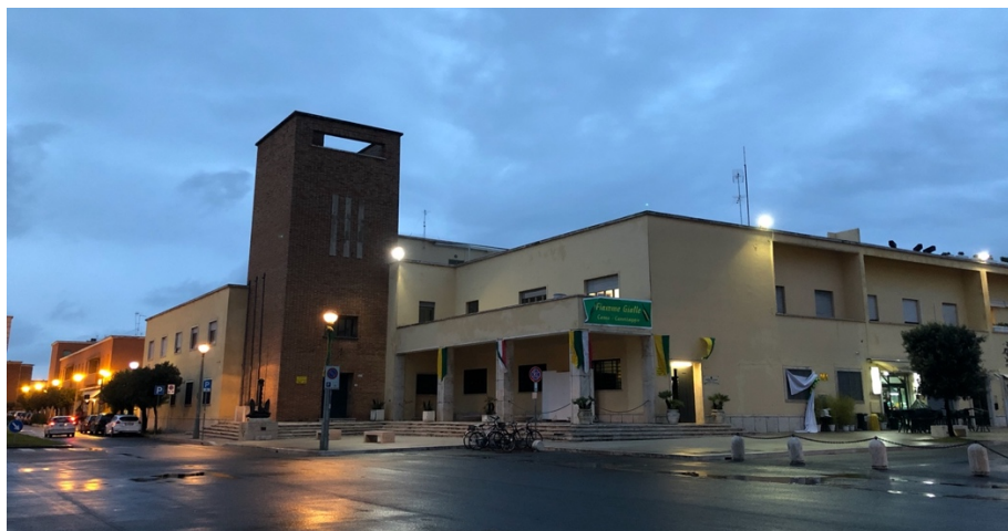
Figure 26 - The ex CDF now Guardia di Finanza headquarter. Source: photo of the author.
