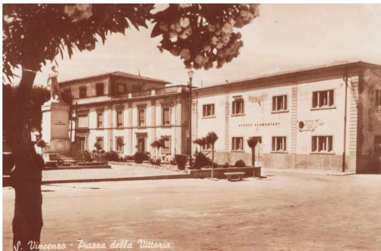
Figure 92 - The ex-CDF of San Vincenzo as an elementary school. Source: http://san-vincenzo-foto-storiche.blogspot.com/2009/09/170-piazze-centrali-20.html
