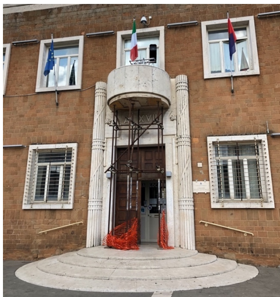
Figure 47 - The ex-CDF now Polizia headquarter. The entrance. Source: photo of the author.
