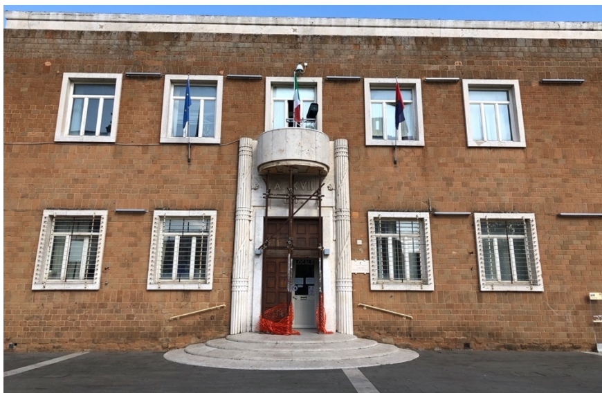
Figure 48 - The ex-CDF now Polizia headquarter. The entrance. Source: photo of the author.
