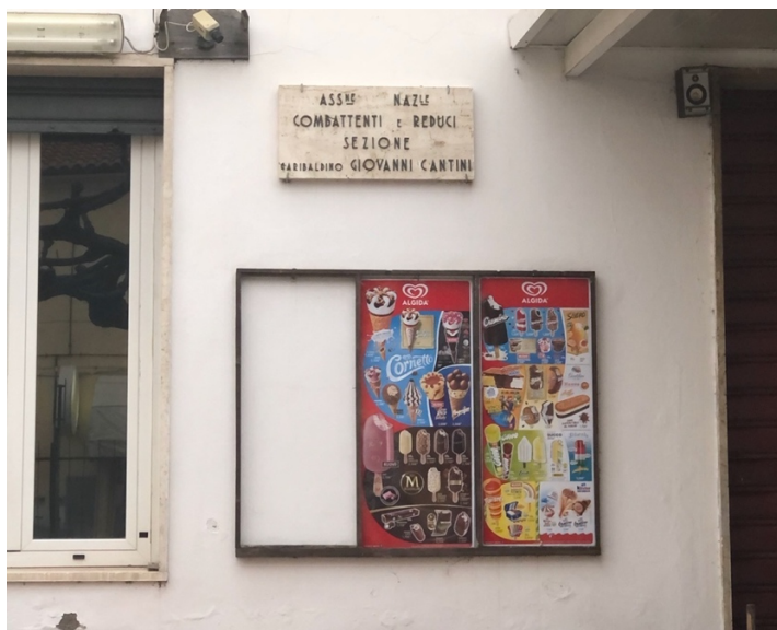
Figure 83 - The plaque on the ex-CDF in San Pietro in Palazzi. Source: photo of the author.
