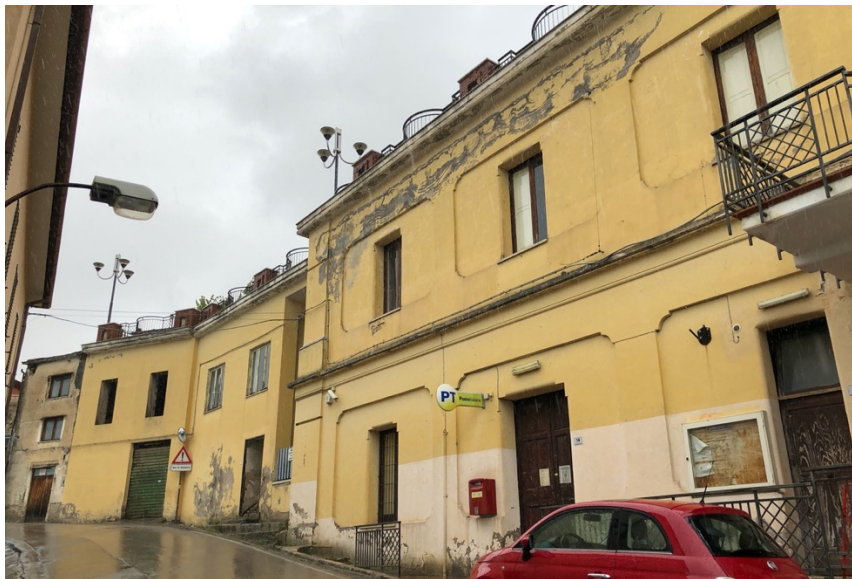
Figure 54 - The ex-CDF now Poste. Source: photo of the author.
