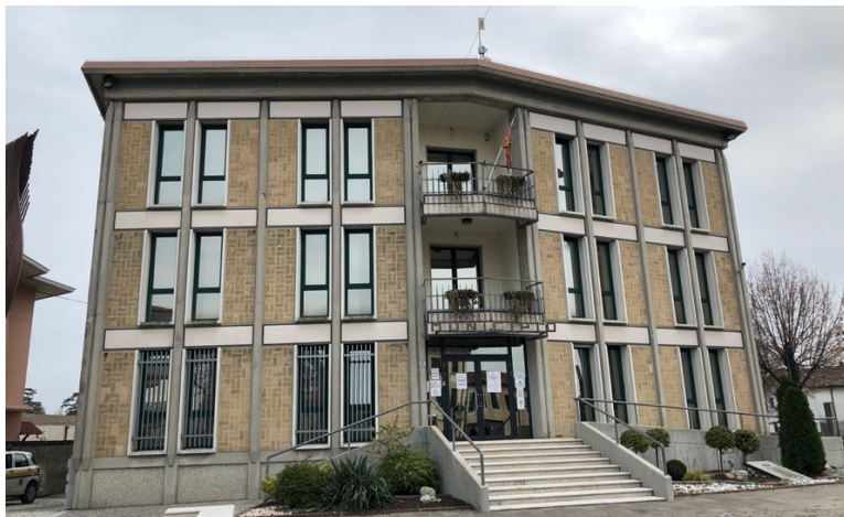
Figure 108 - The ex-CDF, now Municipality. Source: photo of the author.
