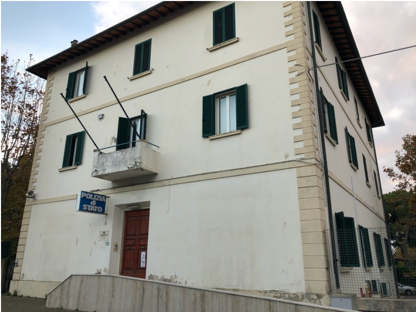
Figure 81 - The ex-CDF in Rosignano Solvay, now a police station. Source: photo of the author.
