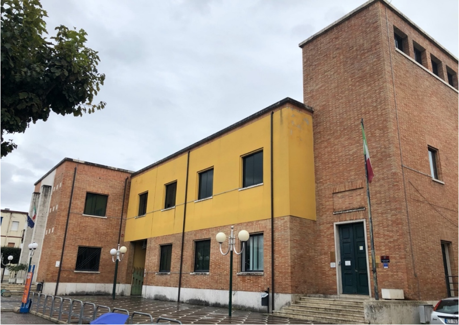
Figure 40 - The ex-CDF of Pontinia. View of the entire building. Source: photo of the author.
