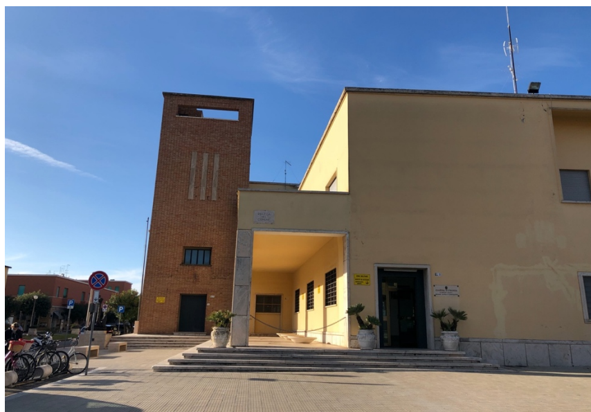
Figure 27 - The ex CDF now Guardia di Finanza headquarter. Side view. Source: photo of the author.
